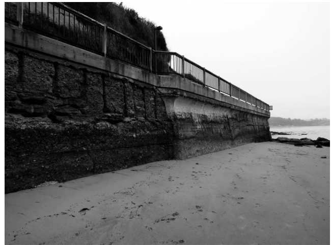
Figure 5. This masonry seawall in Capitola, constructed in the 1930s, is still functioning today.
