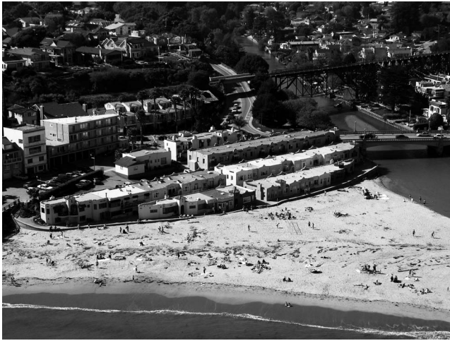
Figure 6. The Venetian Court condominiums, built essentially on the beach in Capitola in 1923, are repeatedly flooded by the combination of storm waves and high tides.
