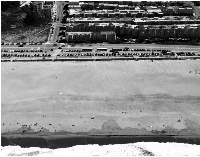
Figure 4. The O'Shaughnessy Seawall along San Francisco's Ocean Beach is one of the oldest in California and was designed and built to withstand every potential type of failure. (Photo courtesy of Kenneth and Gabrielle Adelman, California Coastal Records Project.)
