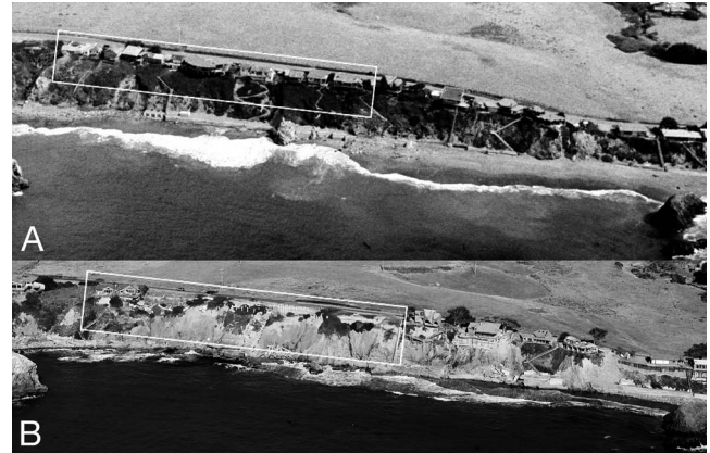
Figure 12. (A) Gleason Beach, Sonoma County coast, in 1979. This group of 21 homes was built on a narrow strip of land adjacent to State Highway 1 on one side and a steep bluff dropping to the shoreline on the other. Septic tanks were placed behind concrete retaining walls on the beach. (Photo courtesy of Kenneth and Gabrielle Adelman, California Coastal Records Project.) (B) Gleason Beach in 2013. Although just 10 homes remained in 2013, many of these were not safe for habitation because of continuing erosion. By 2018 only few houses remained at both ends of this development, and plans are underway to relocate Highway 1 further inland. (Photo courtesy of Kenneth and Gabrielle Adelman, California Coastal Records Project.)
