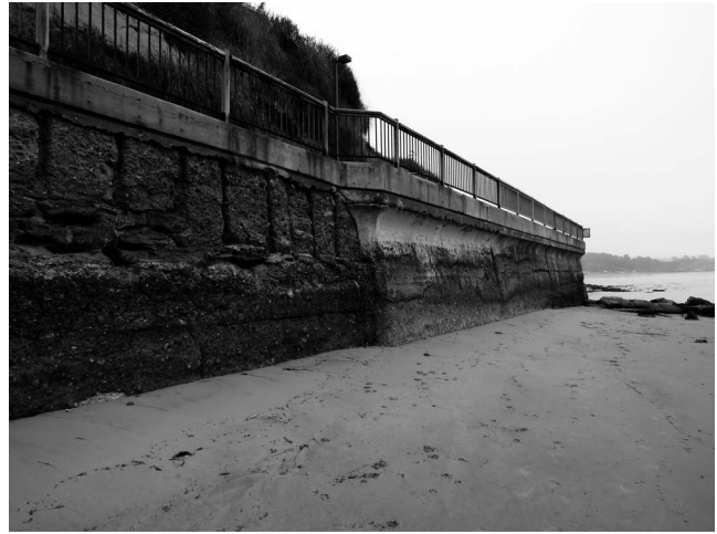
Figure 5. This masonry seawall in Capitola, constructed in the 1930s, is still functioning today.
