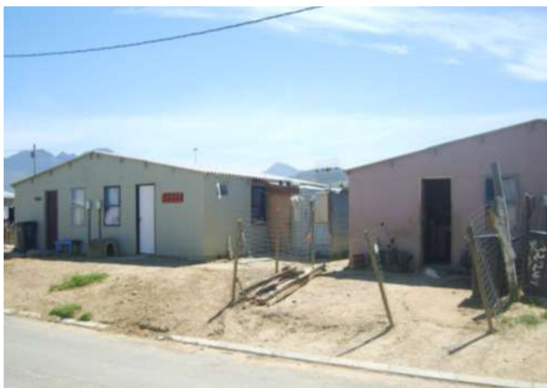
Figure 1. Adjoining shacks in the Greenfields settlement obscuring municipal reticulation systems.
